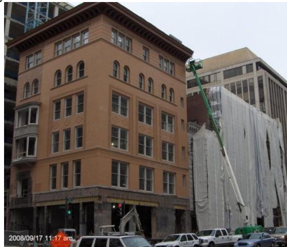
Figure 13 - B&W Building Brick Façade
