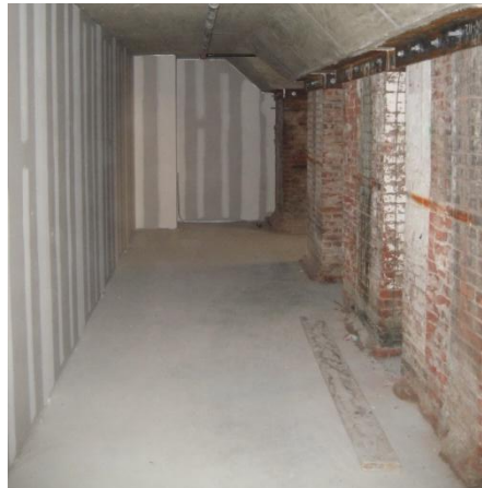
Figure 25 - BW Bldg - B1 Level - Southern View
