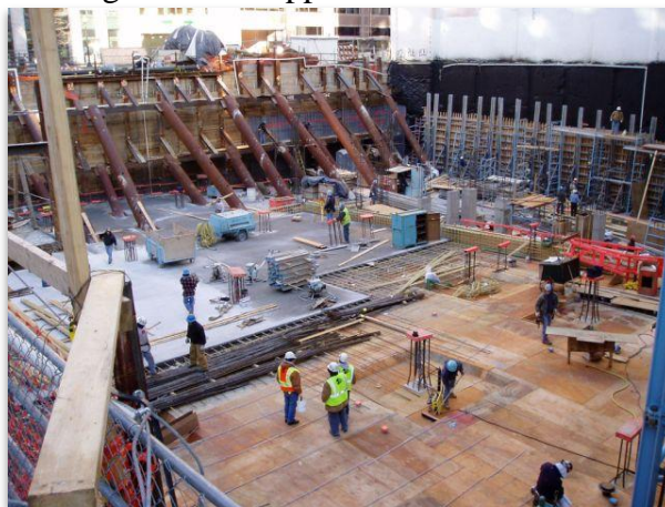
Figure 3 – Excavation Support
