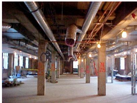
Figure 38 - Bulkhead Housing FPIUs (3)
