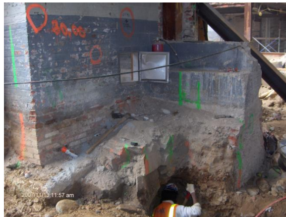
Figure 17 - Nordlinger Underpinning
