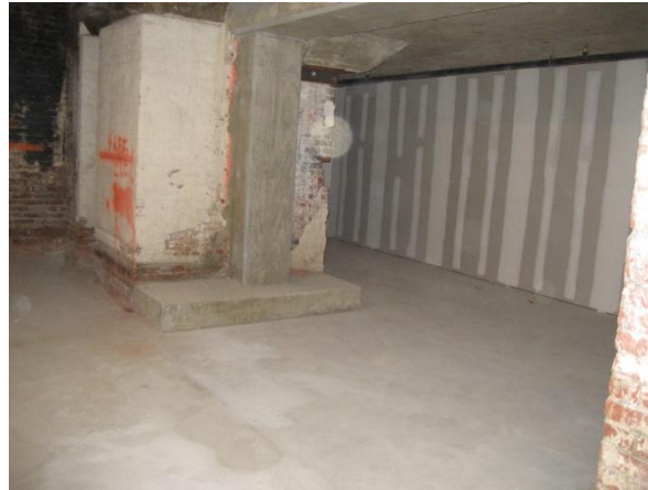
Figure 26 - BW Bldg - B1 Level - East View
