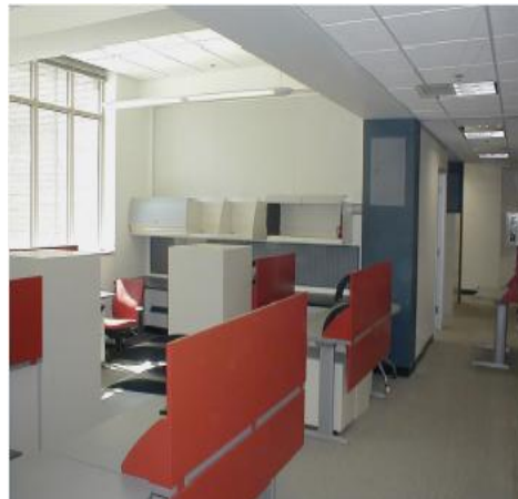
Figure 36 - Bulkhead Housing FPIUs (1)
